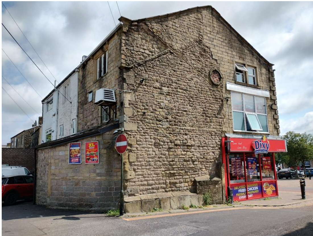
Figure 27 Market Street with evidence of an earlier building and weavers window to the rear
