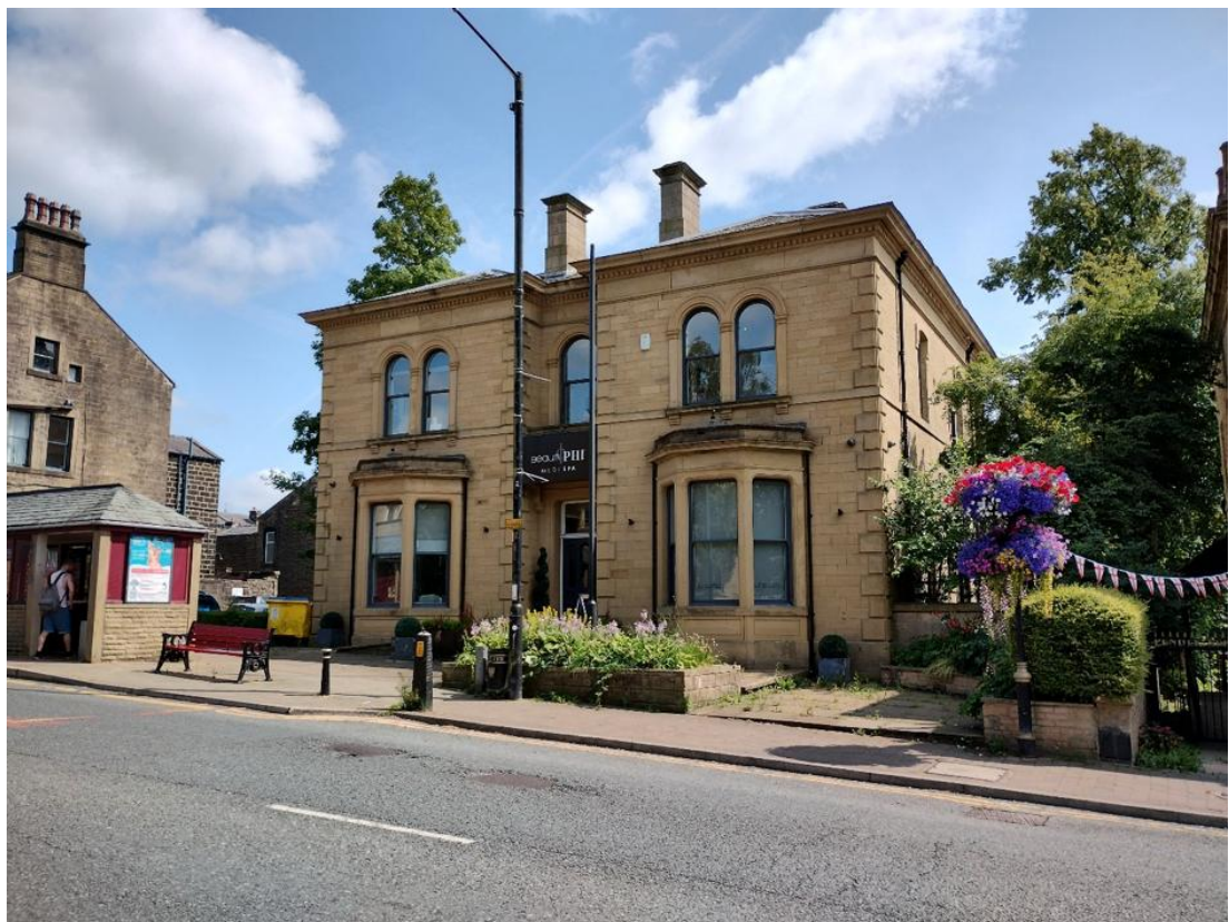
Figure 8 Stanley Villa, 61 Albert Road
