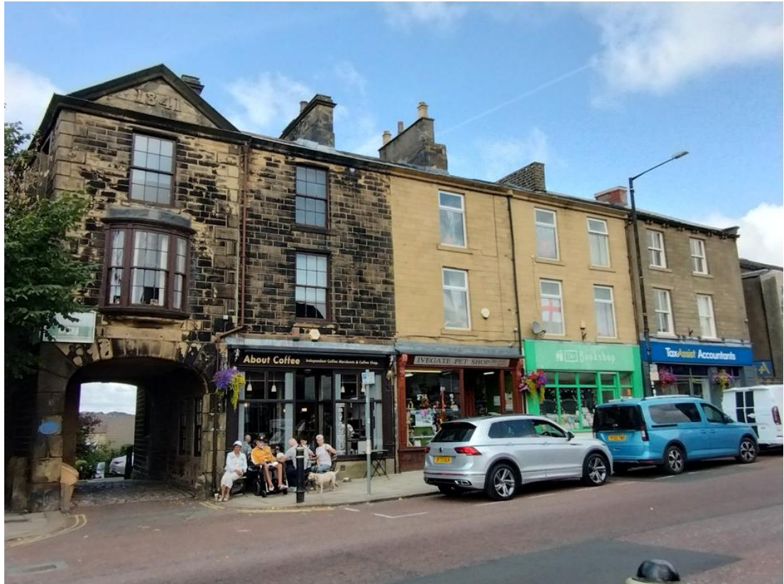
Figure 7 Early Victorian town houses at Ivegate and Market Street
