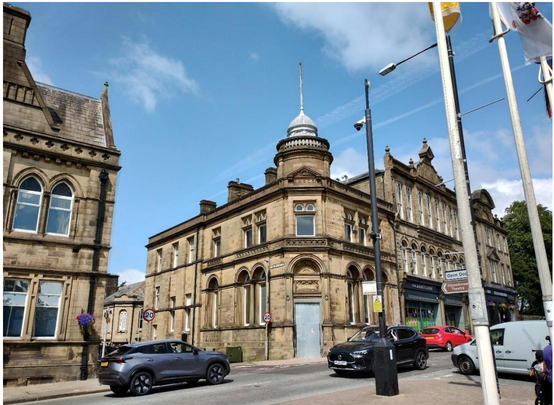
Figure 3 Albert Road with the Town Hall (left), 34 Albert Road and Shakleton Hall
