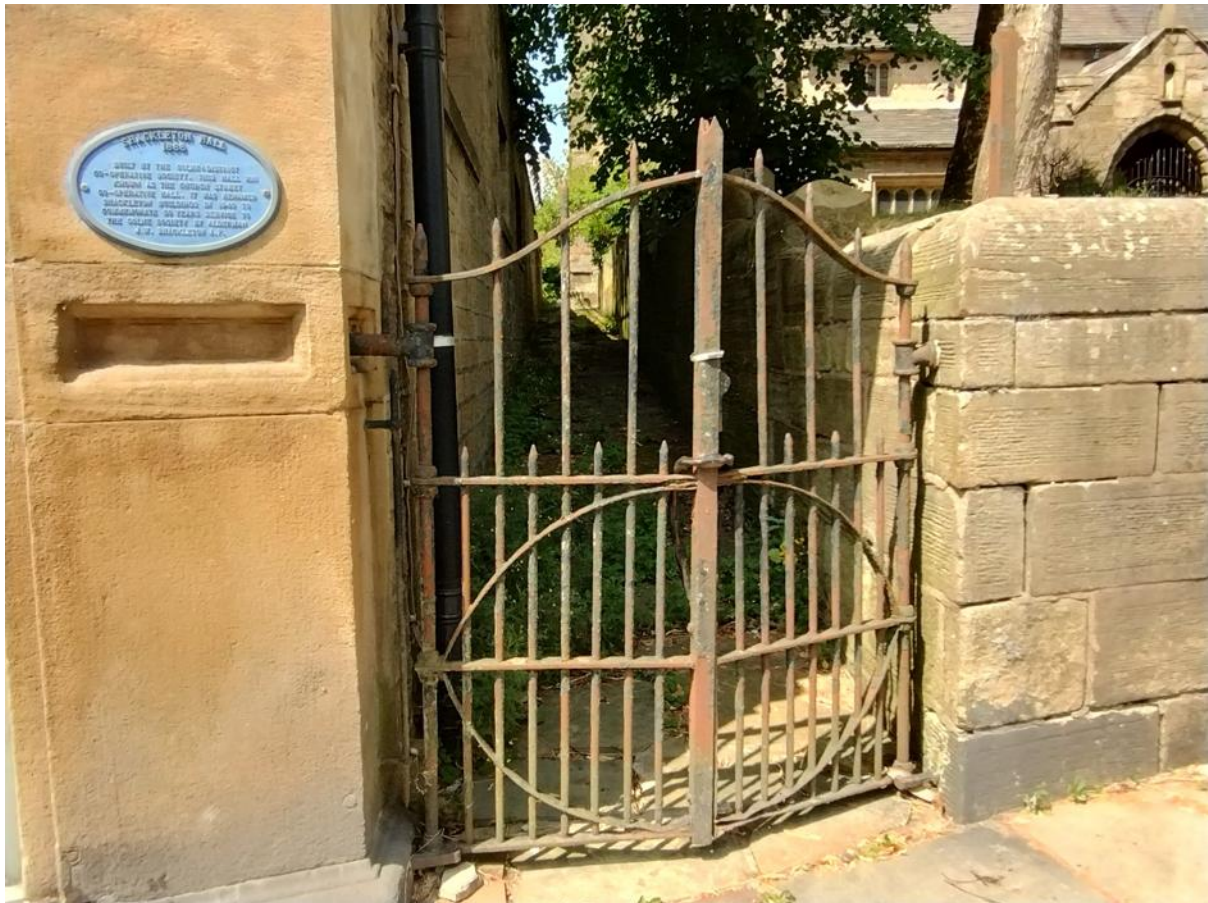
Figure 25 The wrought and cast iron railings to the west of the churchyard
