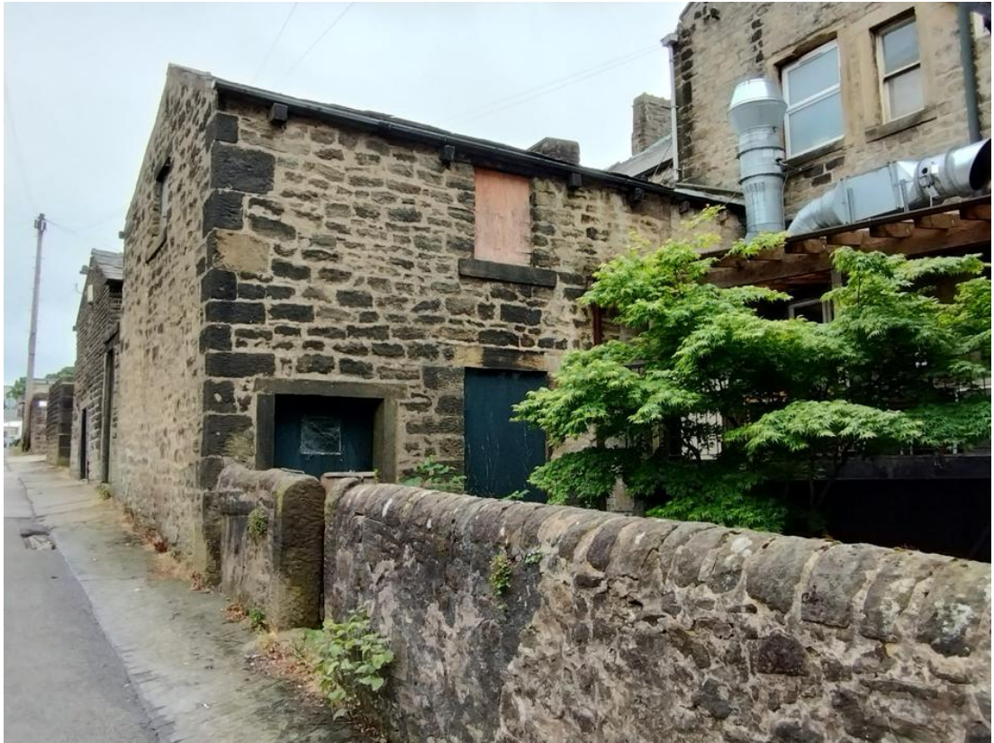
Figure 5 Well-preserved outbuildings to the rear of the Crown Hotel
