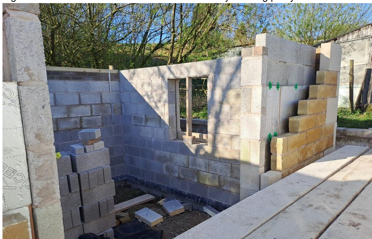
Fig 1.0 Enforcement Visit Photo 07/04/2026 – Utility Building partly erected
