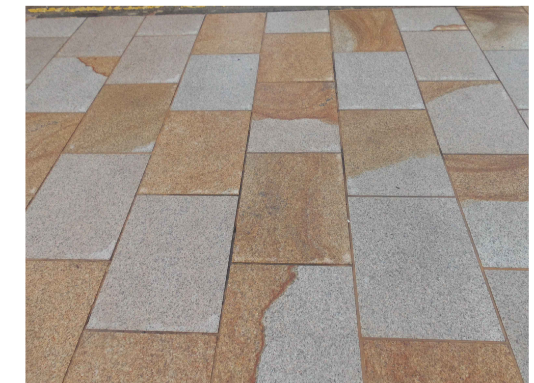
Granite flags specified for works.
