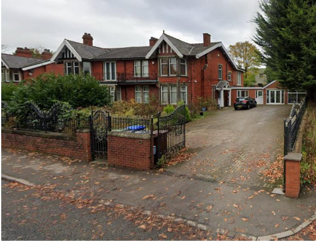
Fig 1.0 Image from Google Street View dated October 2024 (above), prior to installation of boarding to the inside of the railings. There is visibility into the front garden area of the dwelling which allows visibility of the grand red brick dwelling set back from the roadside, which contributes positively to the character and appearance of the area.
