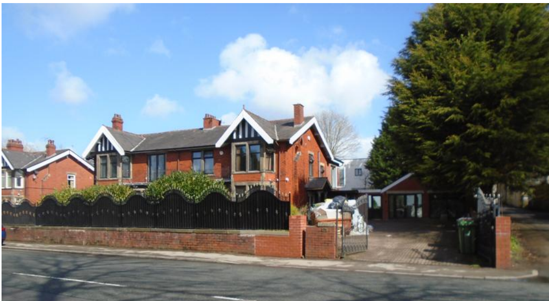
Fig 1.1 Site visit photo: April 2026 (above) with black boarding to the inside of the railings, sitting on top of the red brick wall, creating a dark, overwhelming fortified structure on the edge of the public highway which does not contribute positively to the wider visual amenity.
