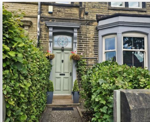
Mix of uPVC windows and doors, with some more sensitive timber framed windows and doors, including sliding sash windows.
