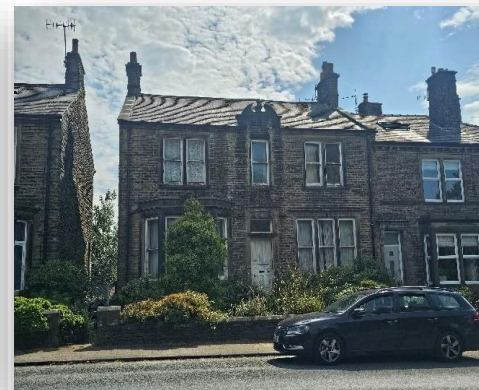
Mix of uPVC windows and doors, with some more sensitive timber framed windows and doors, including sliding sash windows.
