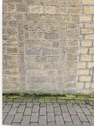
Infilling of original historic features disrupting repetitive features, some of which are unsympathetic
