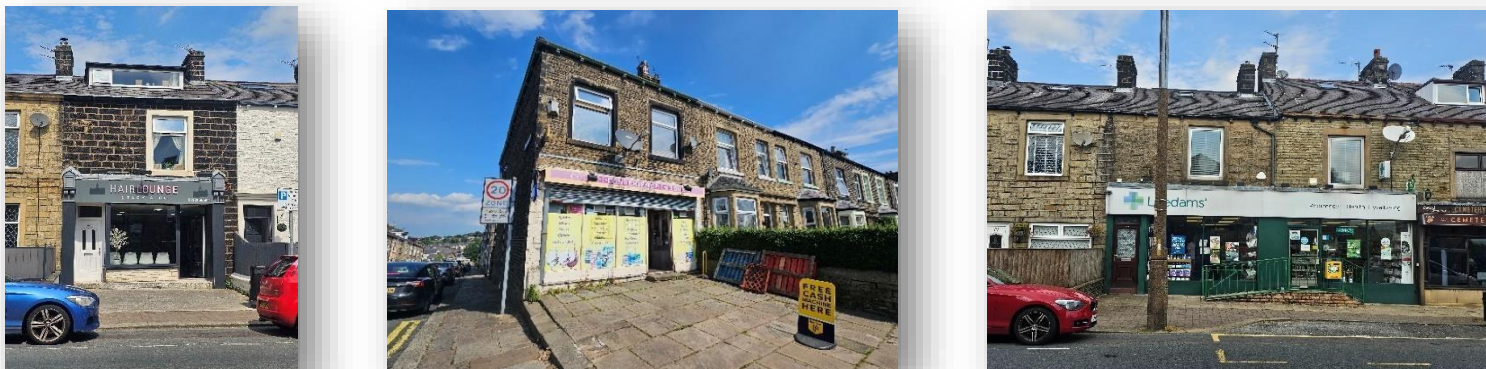
Modern Shopfronts – some with window stickers, posters and advertisements creating visual clutter (centre and right)
