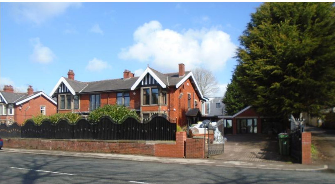
Fig 1.1 Site visit photo: April 2026 (above) with black boarding to the inside of the railings, sitting on top of the red brick wall, creating a dark, overwhelming fortified structure on the edge of the public highway which does not contribute positively to the wider visual amenity.
