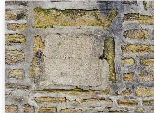
Infilling of original historic features disrupting repetitive features, some of which are unsympathetic
