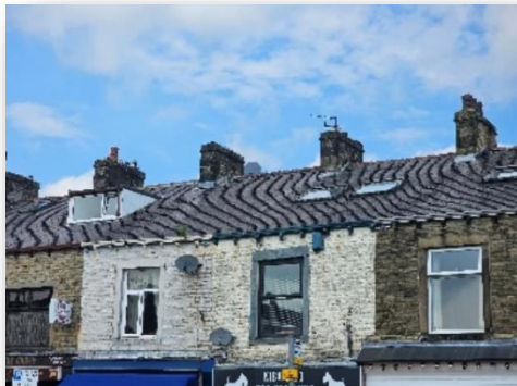
Common issues detracting from the character and appearance of the proposed conservation area, which include modern front facing dormer windows and rooflights, meter boxes, satellite dishes, alarm boxes, security cameras and wiring.
