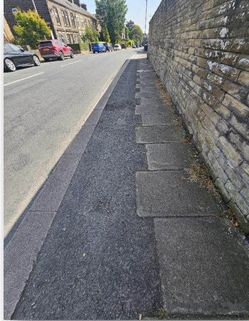
Modern paving similar in size and appearance to historic stone setts (right), tarmac and concrete paving slabs (centre), mix of concrete paving (left)
