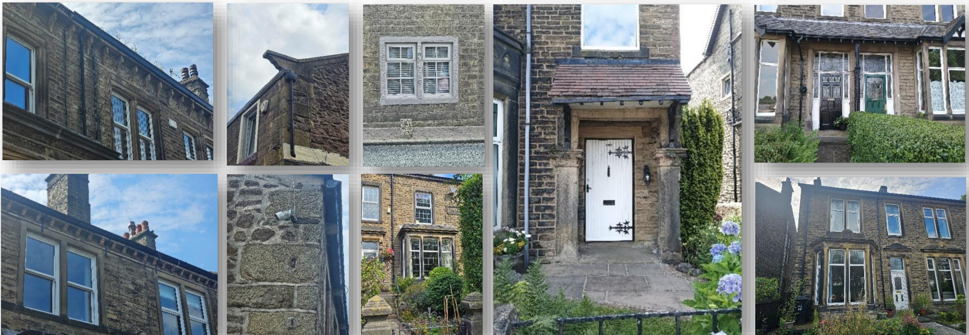
Architectural details (left to right) stone eaves brackets, stone kneeler, stone mullion window, square bay window, entrance porch, continual bay window porch, canted bay window
