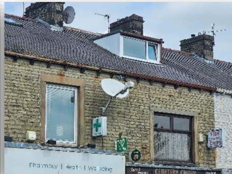
Common issues detracting from the character and appearance of the proposed conservation area, which include modern front facing dormer windows and rooflights, meter boxes, satellite dishes, alarm boxes, security cameras and wiring.
