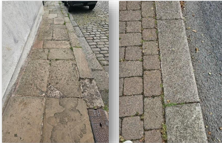
York stone pavement (left) and modern paving and stones (right)
