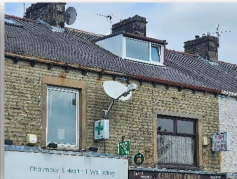
Common issues detracting from the character and appearance of the proposed conservation, which include front facing dormer windows and rooflights, meter boxes, satellite dishes, alarm boxes, security cameras and wiring
