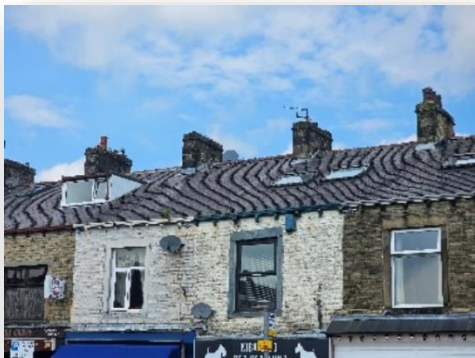
Common issues detracting from the character and appearance of the proposed conservation, which include front facing dormer windows and rooflights, meter boxes, satellite dishes, alarm boxes, security cameras and wiring
