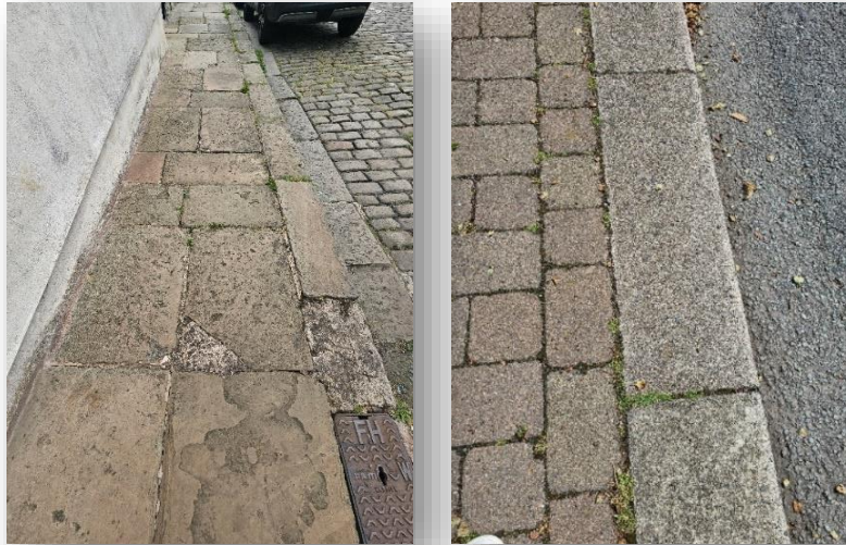
York stone pavement (left) and modern paving and curb stones (right)
