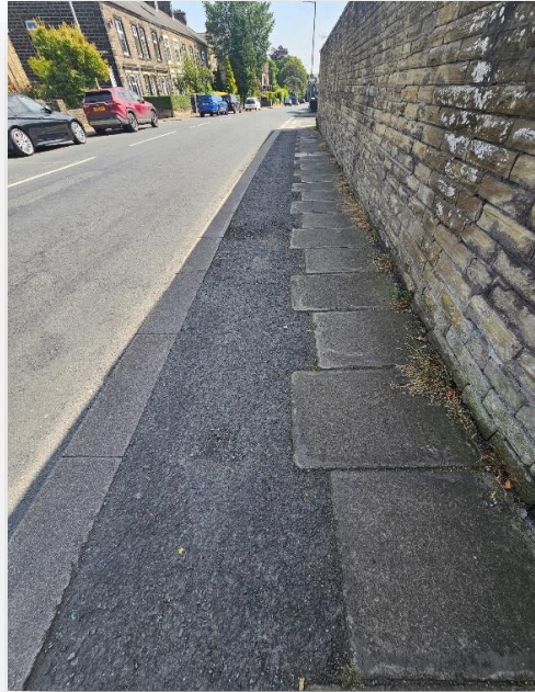
Modern paving stones similar in size and appearance to historic stone setts (right), tarmac and concrete paving slabs (centre), mix of concrete paving (left)
