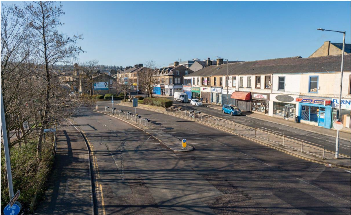
New Scotland Road - existing situation
