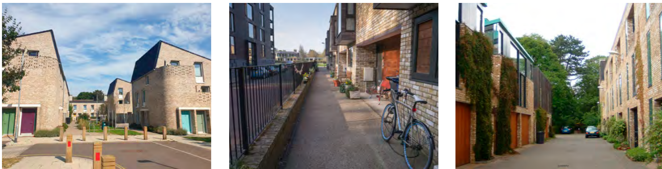
Scale and density of the houses and apartments which could be delivered in the Waterside area. New homes could be designed specifically for multi-generational living or for the elderly, as requested at the consultation.
