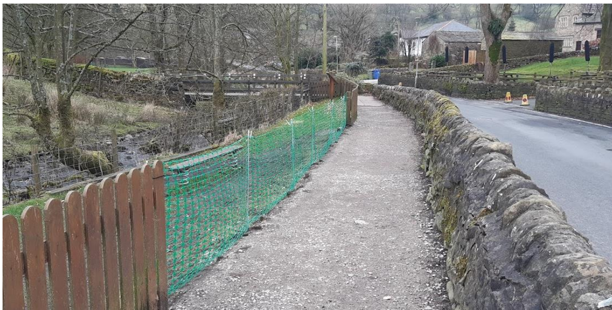
P1 – South Fence - Section Collapsed in February 2024 – All posts were Rotted
