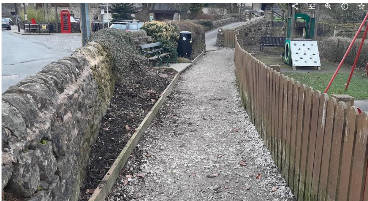
P2– North Fence Section – All posts are loose and horizontal members are rotting
