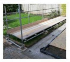
b) for pedestrian-operated plant up to a gross weight of 2t, a proprietary, interlinked ground protection boards placed on top of a compression resistant layer (e.g. 150mm depth of woodchip) laid on a geotextile membrane; Non-slip wearing surface can be installed such as <a href="http://www.ground-quards.co.uk/solutions/tree-root-protection/">http://www.ground-quards.co.uk/solutions/tree-root-protection/</a>
