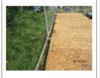
c) for wheeled or tracked construction traffic exceeding 2t gross weight, an alternative system (engineer approved) designed with arboricultural input to accommodate the likely loading to which it will be subjected'
