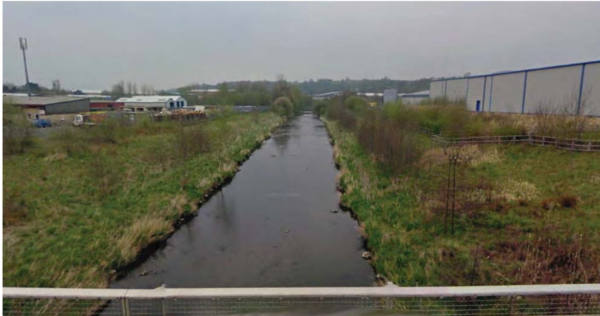
Figure 6.1: Pendle Water Viewed Downstream from Churchill Way
