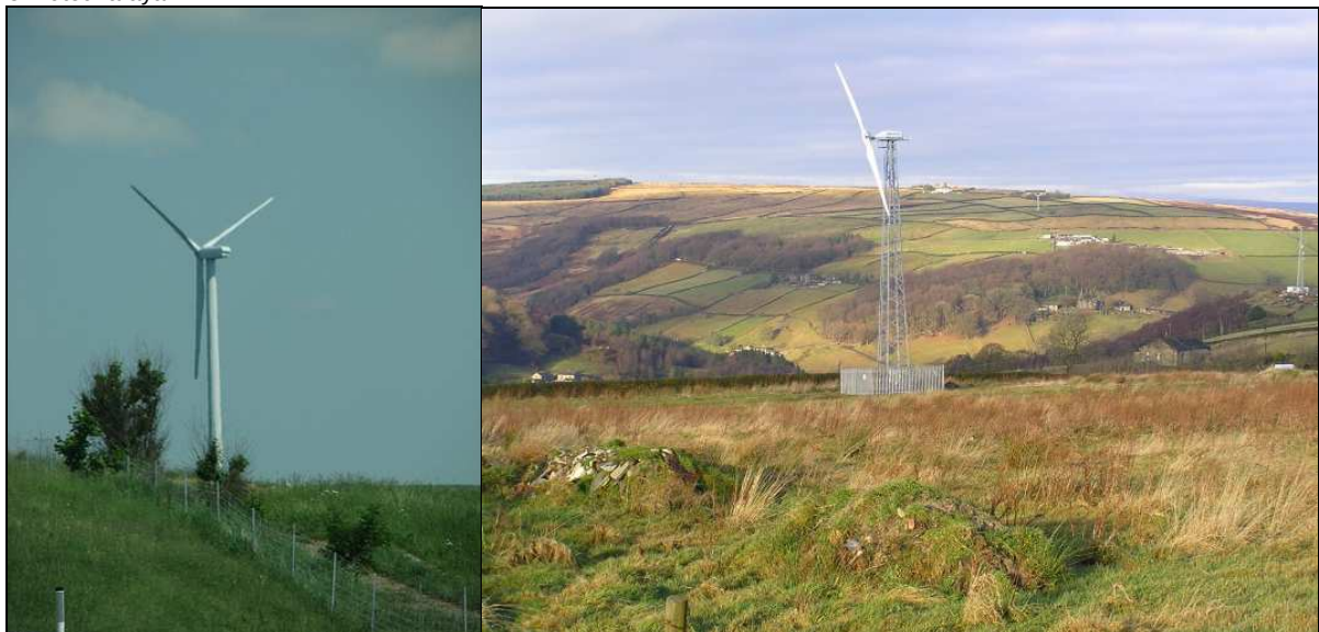
Typical three- and two-bladed turbines
