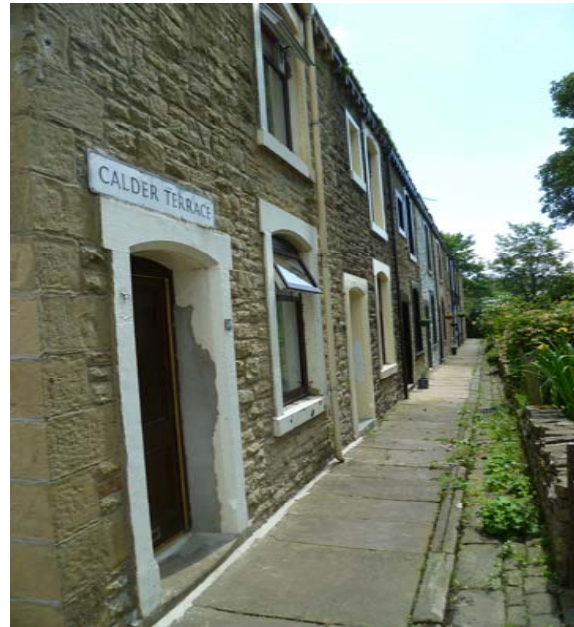
Calder Terrace - sandstone paving flags and kerb edgings
