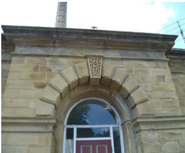
Office range - rusticated arched doorway with keyblock
