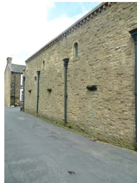
Northern weaving shed wall – stone corbelling to the parapet and round-headed ventilation openings
