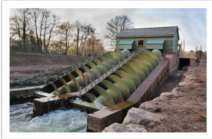
Archimedes-screw micro-hydro turbine, near Monmouth 1
