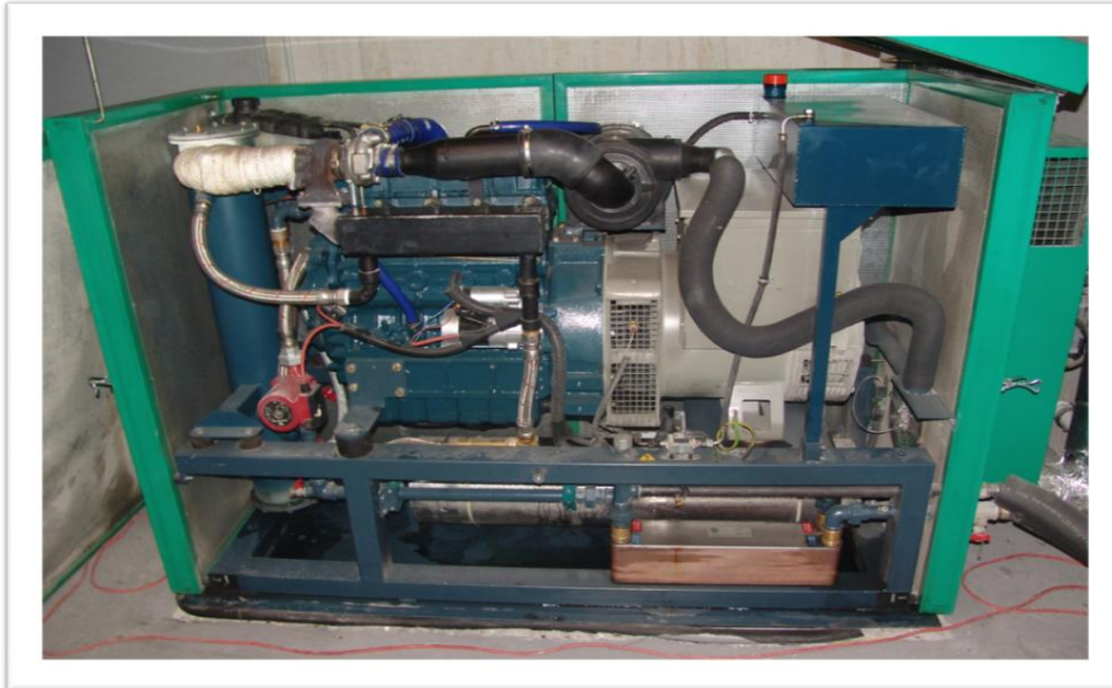
A CHP unit fuelled by oil. Acoustic insulation removed
