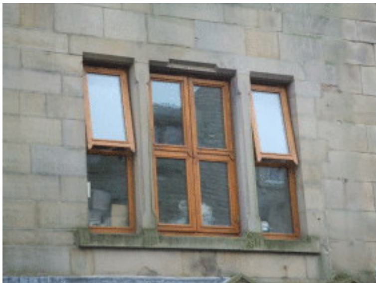
Picture 4.5 The weakened form of most mock sashes and their non-traditional appearance when open can detrimentally affect the character and appearance of a conservation area
