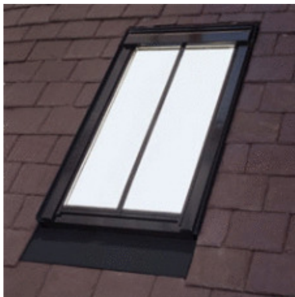
Picture 4.4 A conservation rooflight lies flush with the existing roof
