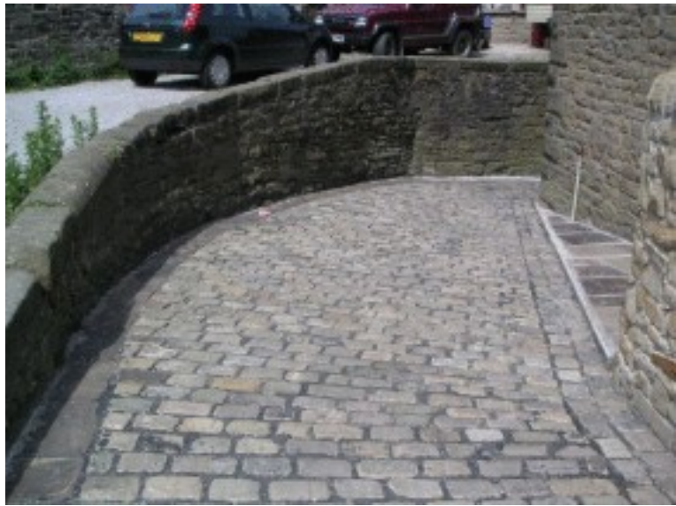
Picture 3.1 Stone setts add greatly to an area's character
