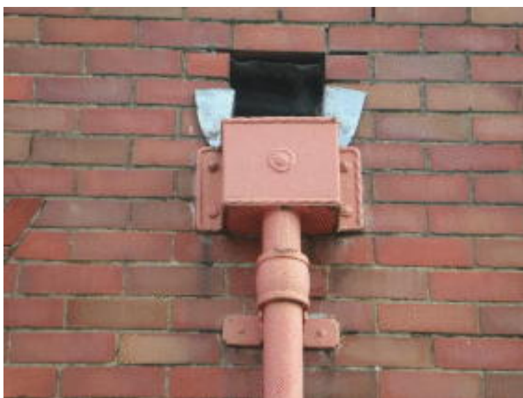
Picture A.3 Detail is 'lost' if the wrong colours are used
