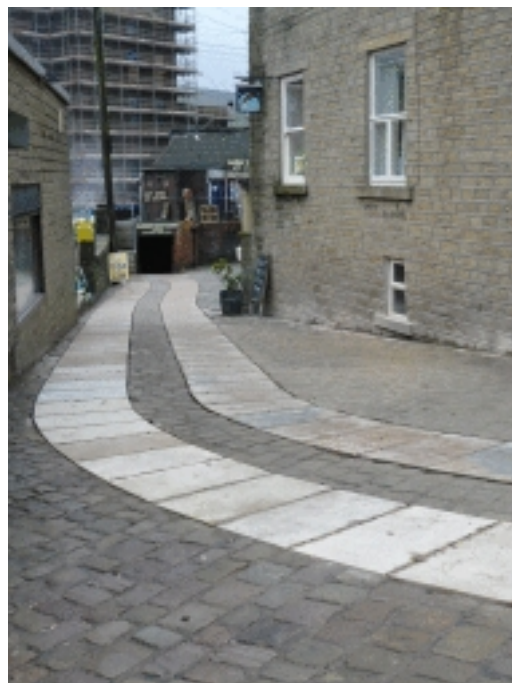
Picture 2.26 Smooth paving provided through a setted area to enable easier access
