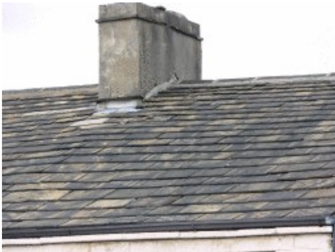
Picture 2.13 Typical example of stone slate roofing
