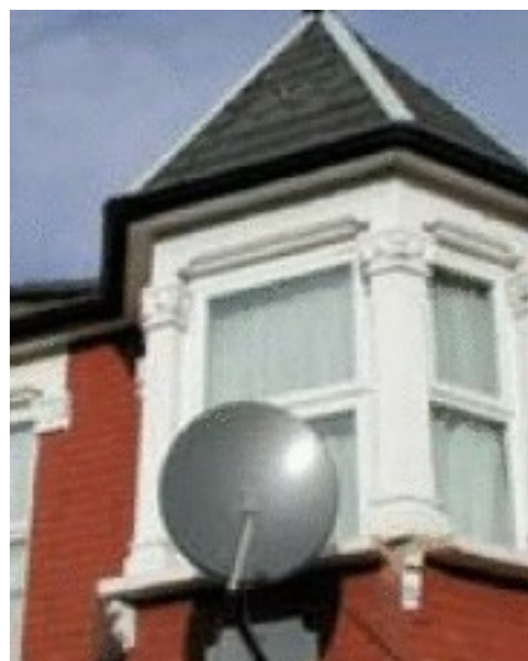
Picture 4.8 Poorly situated satellite dish covering principle features
