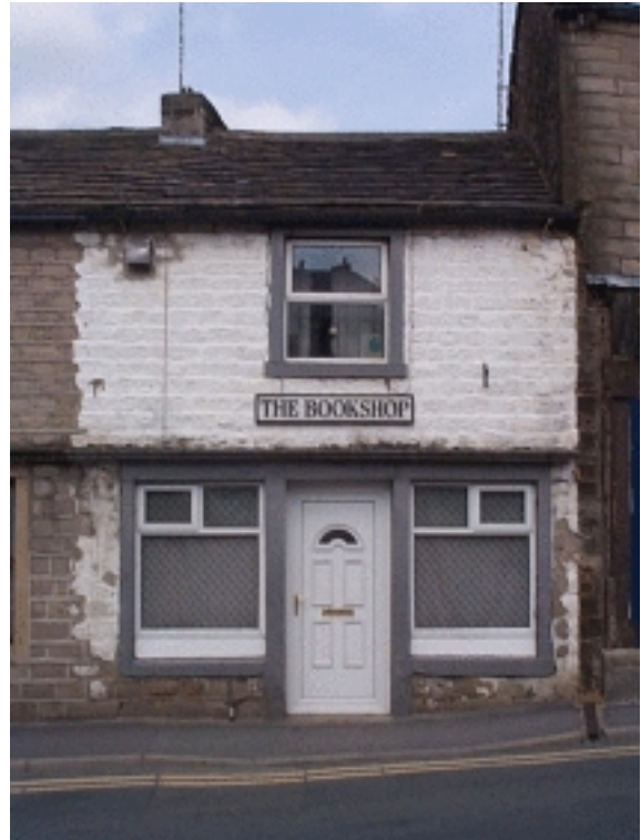
Picture 4.6 New windows and doors in uPVC can damage the character and appearance of buildings
