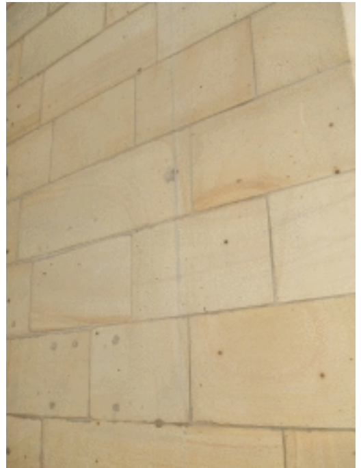
Picture 2.10 Ashlar – blocks of accurately dressed, cut, squared and finished stone forming perfect courses
