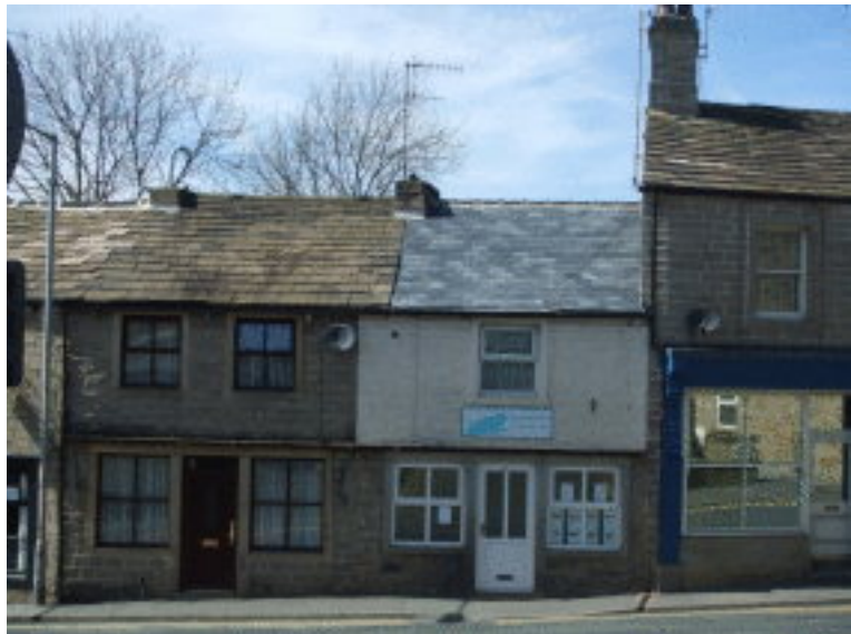
Picture 4.1 The removal and replacement of stone slate can cause harm to the character and appearance of a conservation area especially within a row of similar properties
