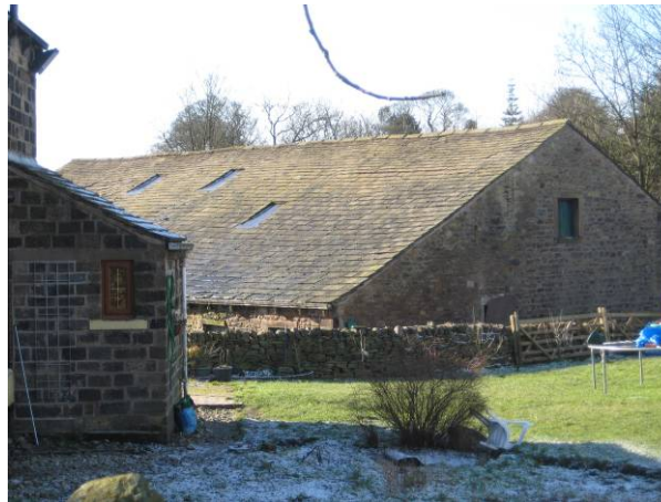
A heavy stone slate roof at Lower Park Hill Farm barn
