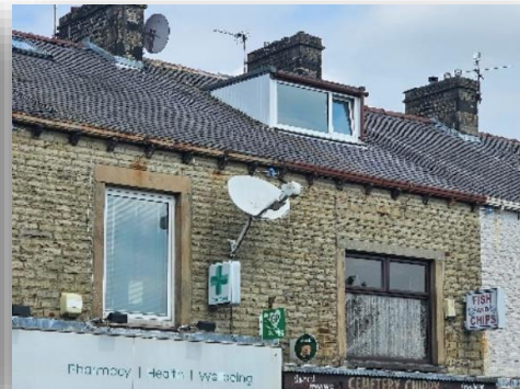
Common issues detracting from the character and appearance of the conservation area, which include modern front facing dormer windows and rooflights, meter boxes, satellite dishes, alarm boxes, security cameras and wiring.
