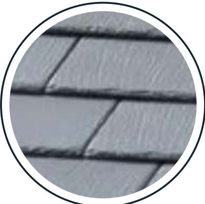
Blue-grey artificial slate roof
