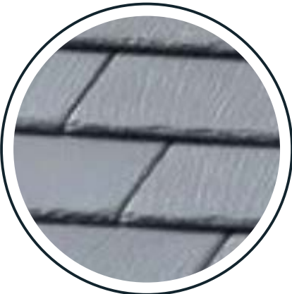
Blue-grey artificial slate roof
