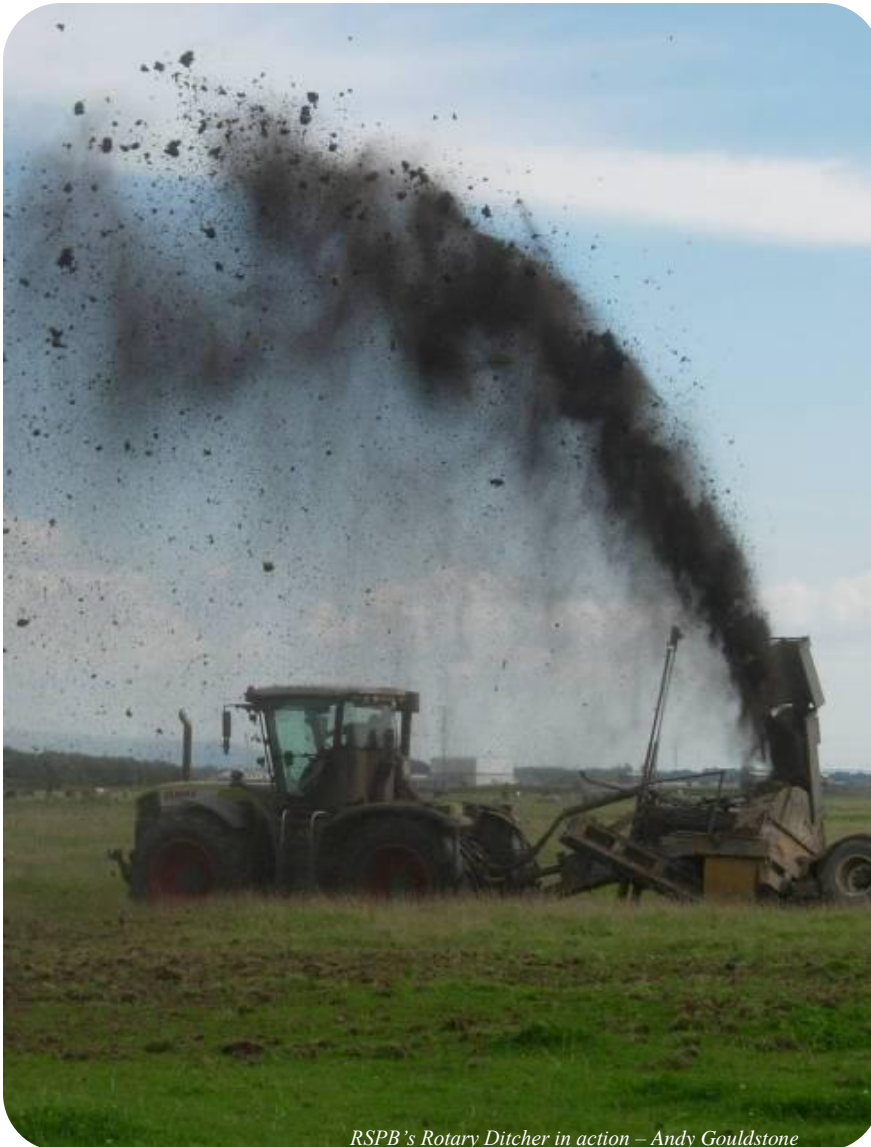
RSPB's Rotary Ditcher in action – Andy Gouldstone
