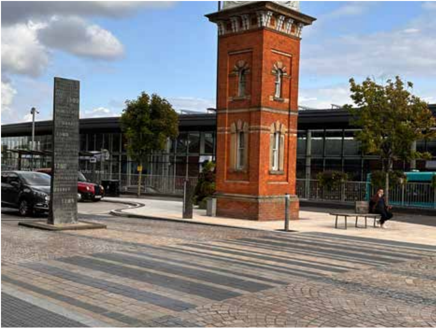
Stamford New Road in Altrincham, where high quality public realm works have redefined the highway space, permitting access and parking for cars as well as loading for shops, but prioritising the experience for pedestrians first. Combination of different paving material within the carriageway, visually narrows it and helps to calm traffic speeds, without reducing the width of the road space.
