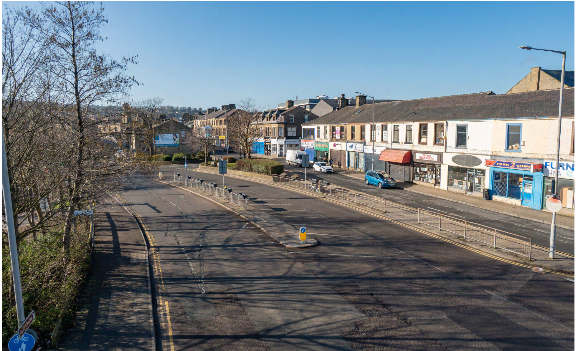
New Scotland Road - existing situation
