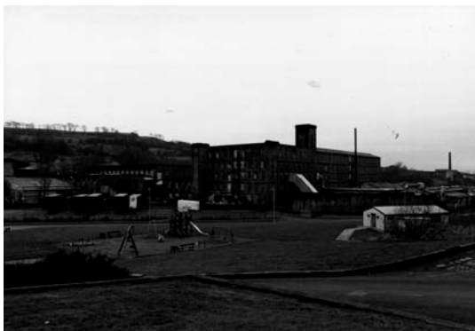
The spinning mill, south weaving shed and offices
