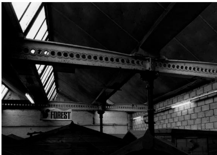
Fig 7. Interior of Primet Mill, Colne, showing cast-iron columns and bridging beams. (NMR: MF98/02788/04A)
