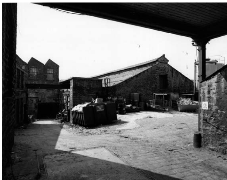
Fig 21. Foundry building of 1861 at Primet Foundry, Colne. (NMR: AA99/03967).
