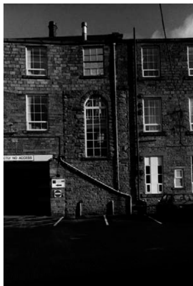
Fig 23. Beam-engine house at Lomeshaye Mills, Nelson. (NMR: MF98/01720/19)
