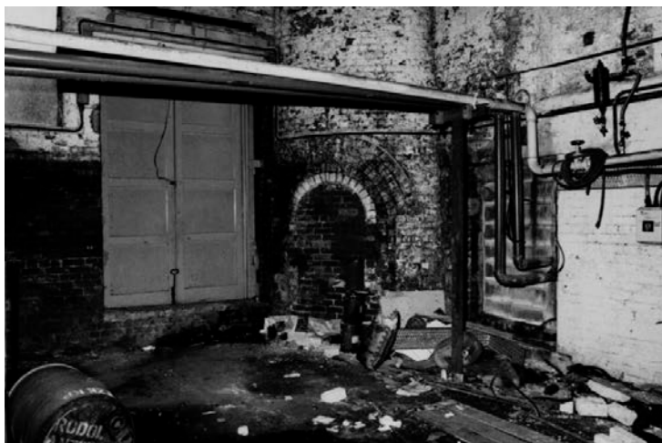
Fig 25. Base of the chimney at Holmefield Mills, Barrowford, showing the opening for the boiler flue. (NMR: 301/U/3A)
