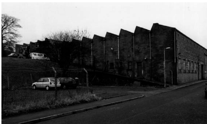
Fig 6. Bankfield Mill, Colne. (NMR: MF98/02787/23)
