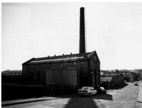
Fig 13. Brook Shed, Earby. (NMR: AA99/03992)
