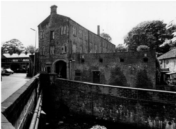
Fig 5. Higherford Mill, Higherford. (NMR: AA99/03949)
