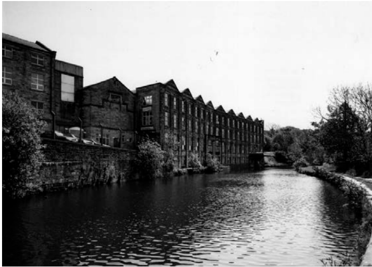
Fig 8. Lob Lane Shed, Brierfield. (NMR: AA99/03979)
