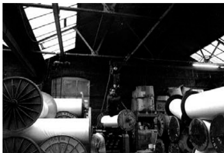
Fig 15. Boundary Mill, Nelson. Interior of 1950's extension showing warp beams and the original exterior wall. (NMR: MF98/01721/22)
