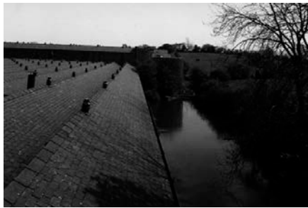
Fig 28. The lodge at Fernbank Shed, Barnoldswick. (NMR: MF98/02795/23)
