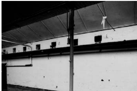
Fig 26 (above). Weaving shed wall at Holmefield Mills, Barrowford, showing wall boxes for line shafts. (NMR: 301U/21A).
