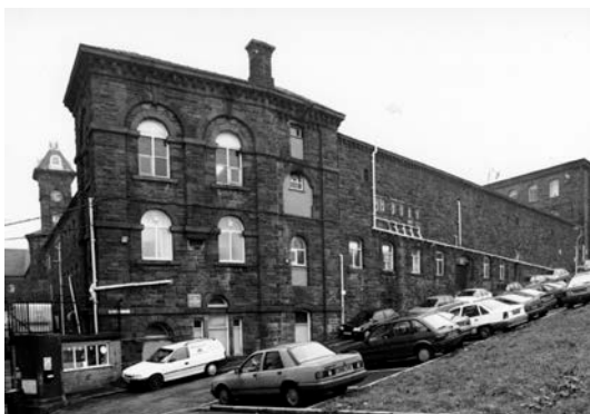
South-east weaving shed and warehouses
