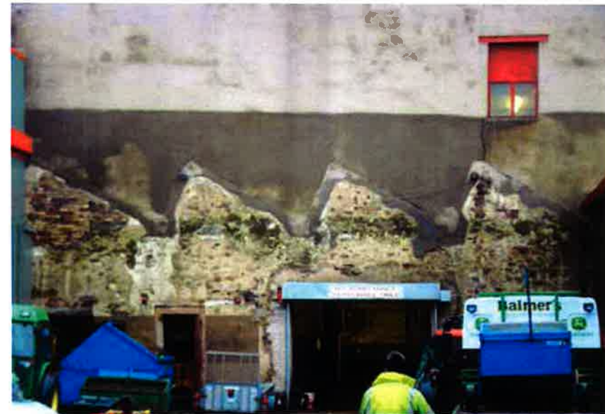
029: Only the scar from the saw-tooth roof remains of this demolished weaving shed near Belle Vue Mill, Burnley
