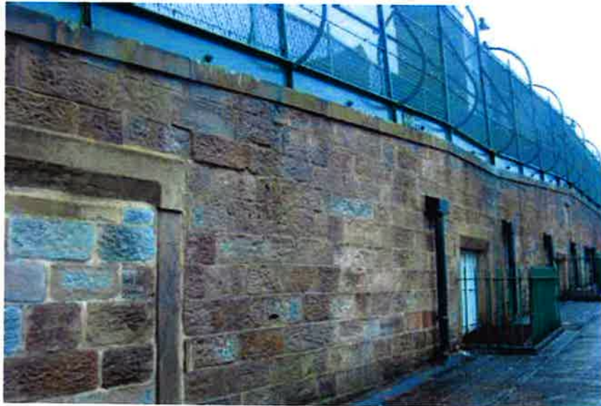
005: Trafalgar Mill, Burnley is terraced and set partially underground
