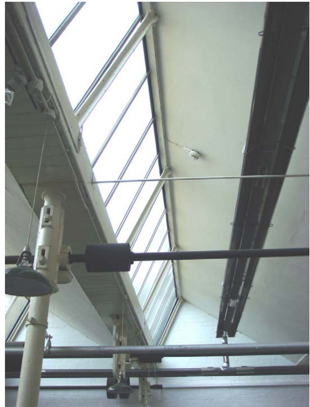
Fig 10. Structure - Internal view of the weaving shed
