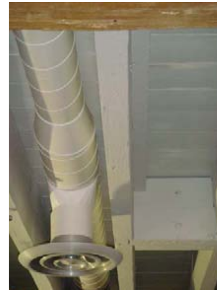
Fig. 33. Warm air ducting
