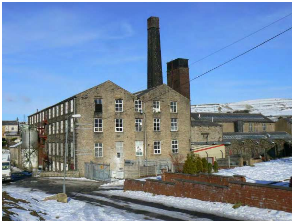
Plate 44: Britannia Mill at Britannia, near Bacup
