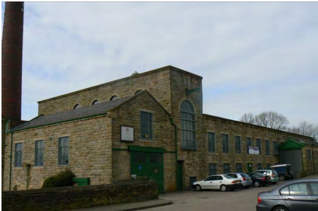
Plate 47: Queen Street Mill, Harle Syke
