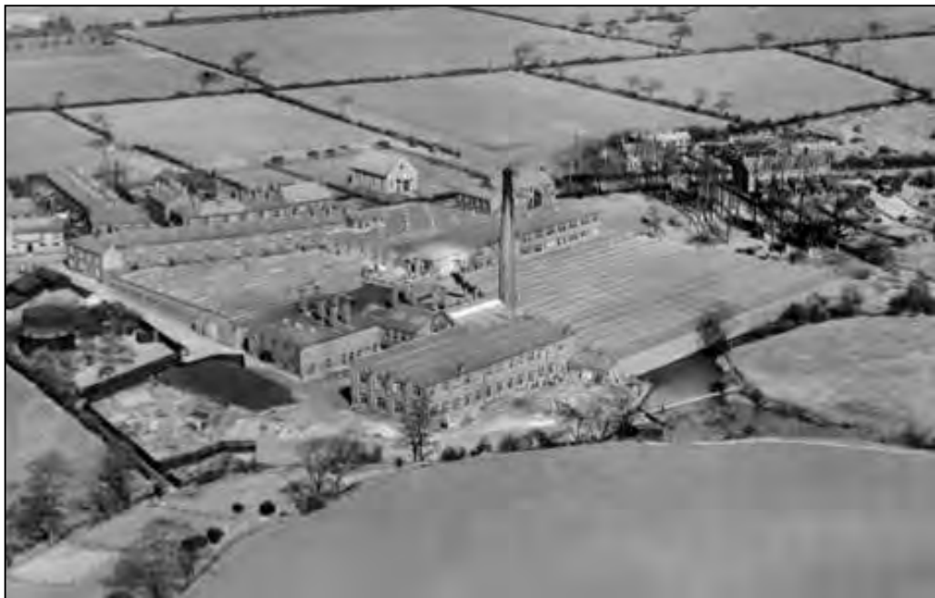
Plate 29: Aerial view of Grove Mill in Eccleston in 1929
