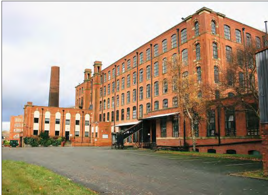
Plate 15: The rear elevation of Centenary Mill in Preston, following its conversion to apartments
