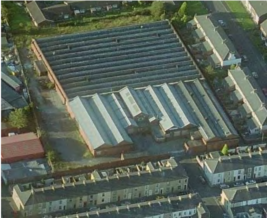
Plate 38: Aerial view of Albert Mill in Rishton
