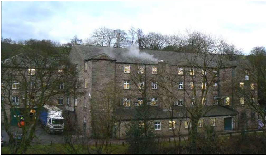
Plate 14: Calder Vale Mill of 1835, in Calder Vale, Wyre
