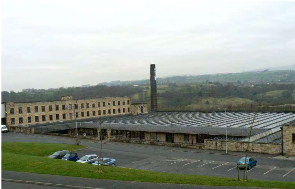
Plate 19: Hollin Bank Mill in Brierfield, refurbished as a retail outlet
