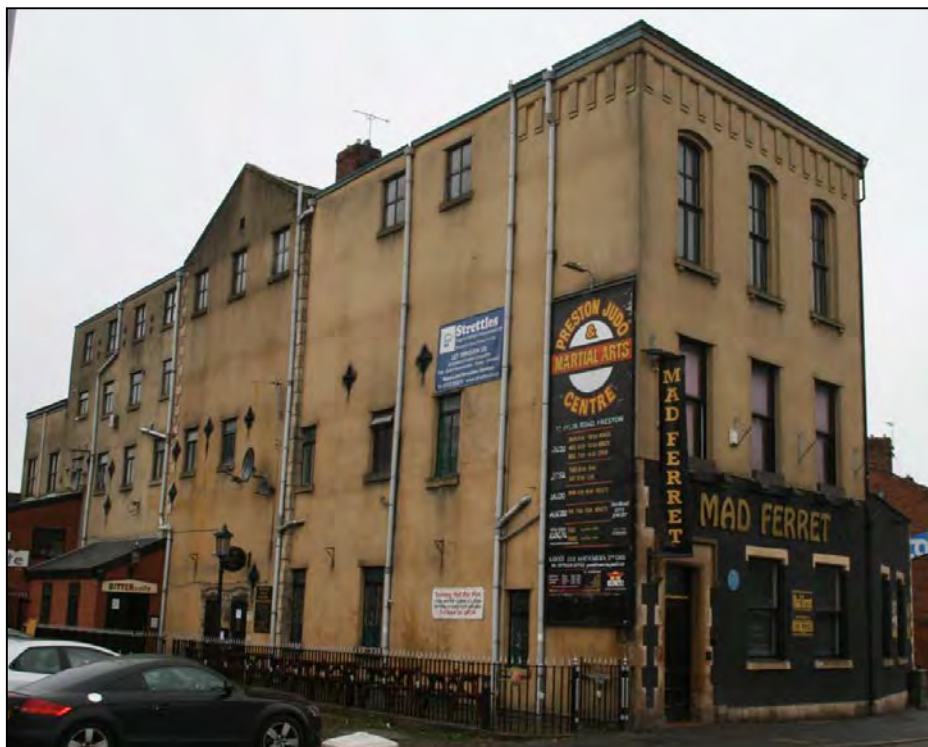
Plate 7: The Grade II-listed Spital's Moss Mill, Preston
