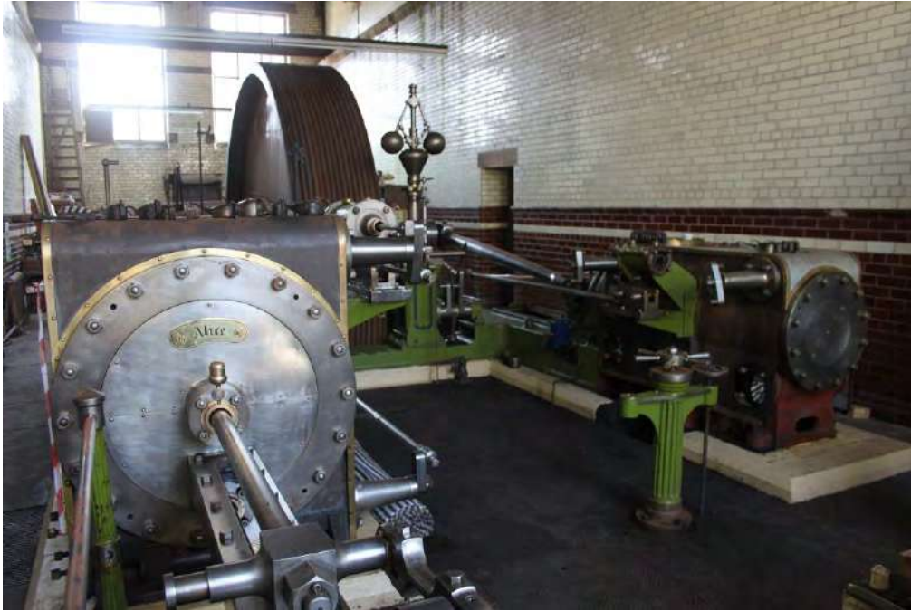
Plate 50: The engine house at Grane Mill, Haslingden
