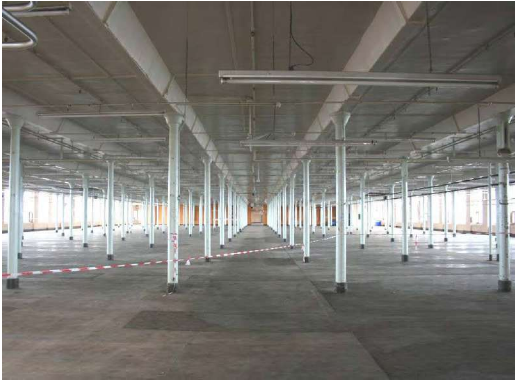
Plate 25: One of the unoccupied floors in Tulketh Mill, Preston
