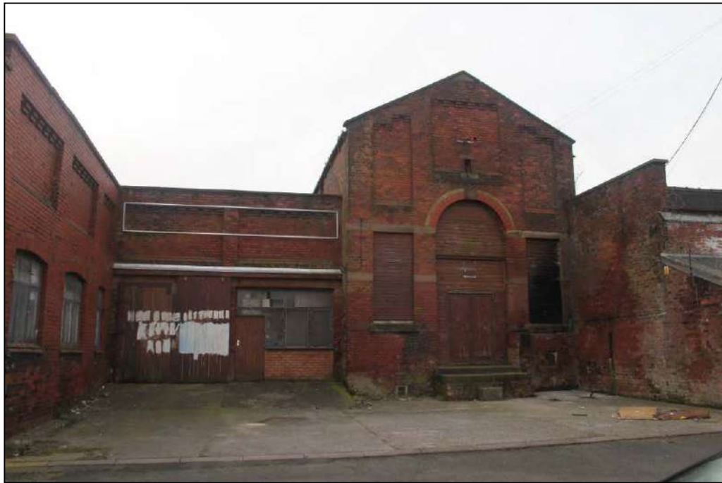
Plate 36: The engine house at Bankfield Mill, Kirkham
