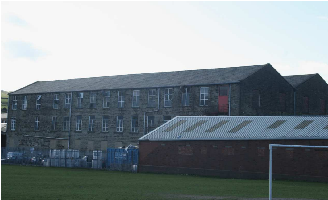
Bridge End Mill
