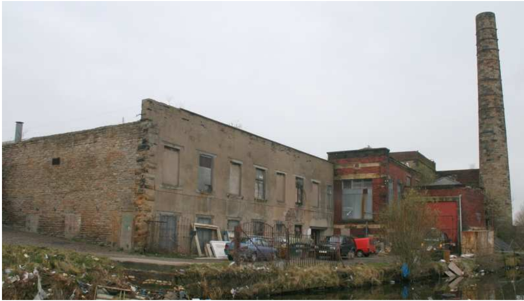
Derelict power plants, and weaving shed with basement, Whittlefield Shed
