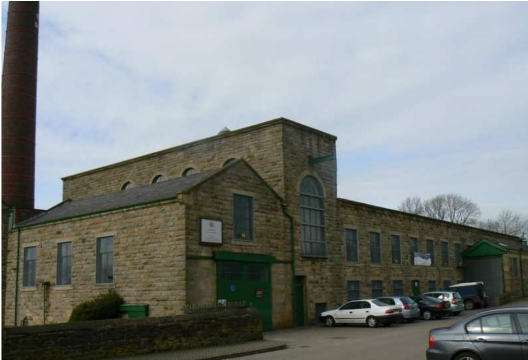
Power complex and weaving shed, Queen Street Mill
