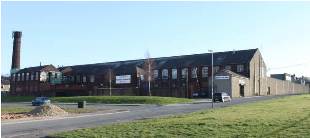
Hargher Clough Mill from the north-west
