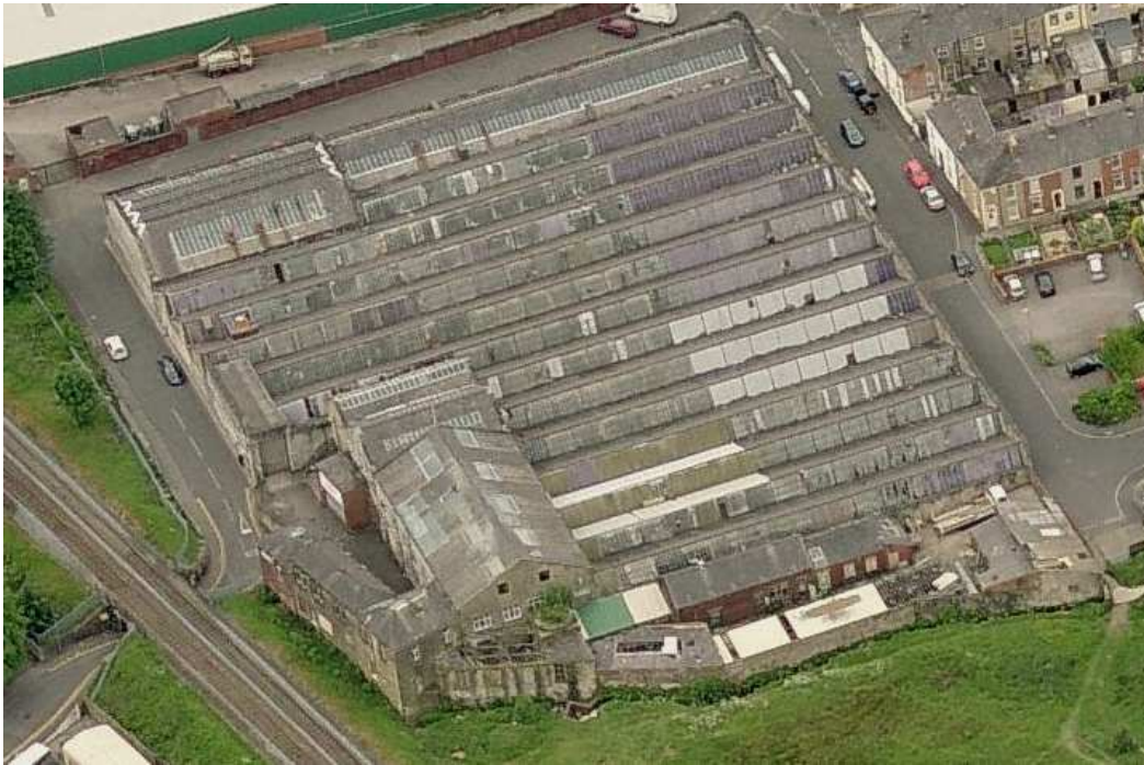
Aerial view of Roe Lee Mill
