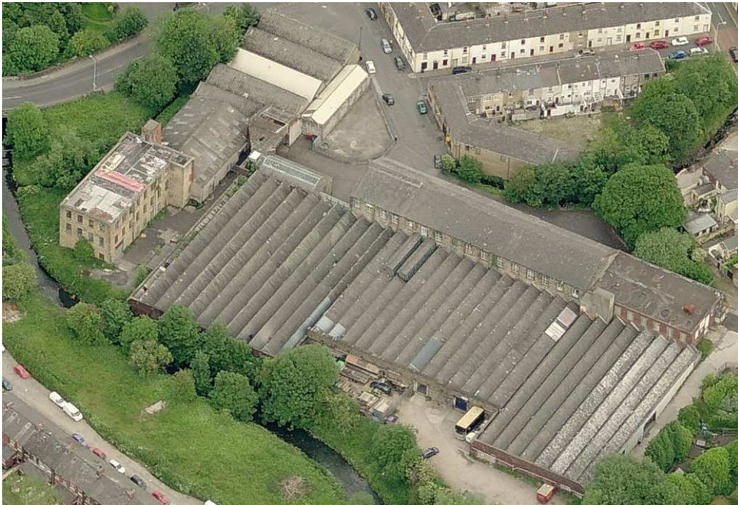
Recent aerial view of Lower Darwen Mill
