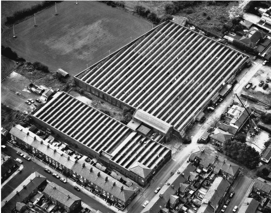
Aerial view of Bankfield Mill taken in 1988
