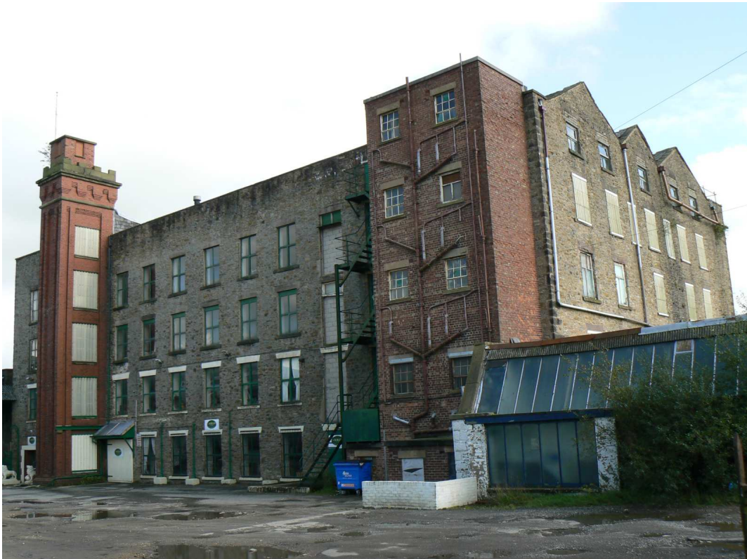
The spinning block and weaving shed of Abbey Mill
