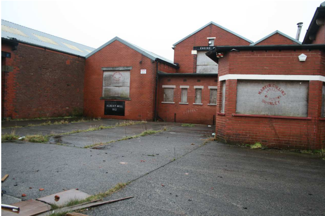
The engine and boiler houses at Albert Mill
