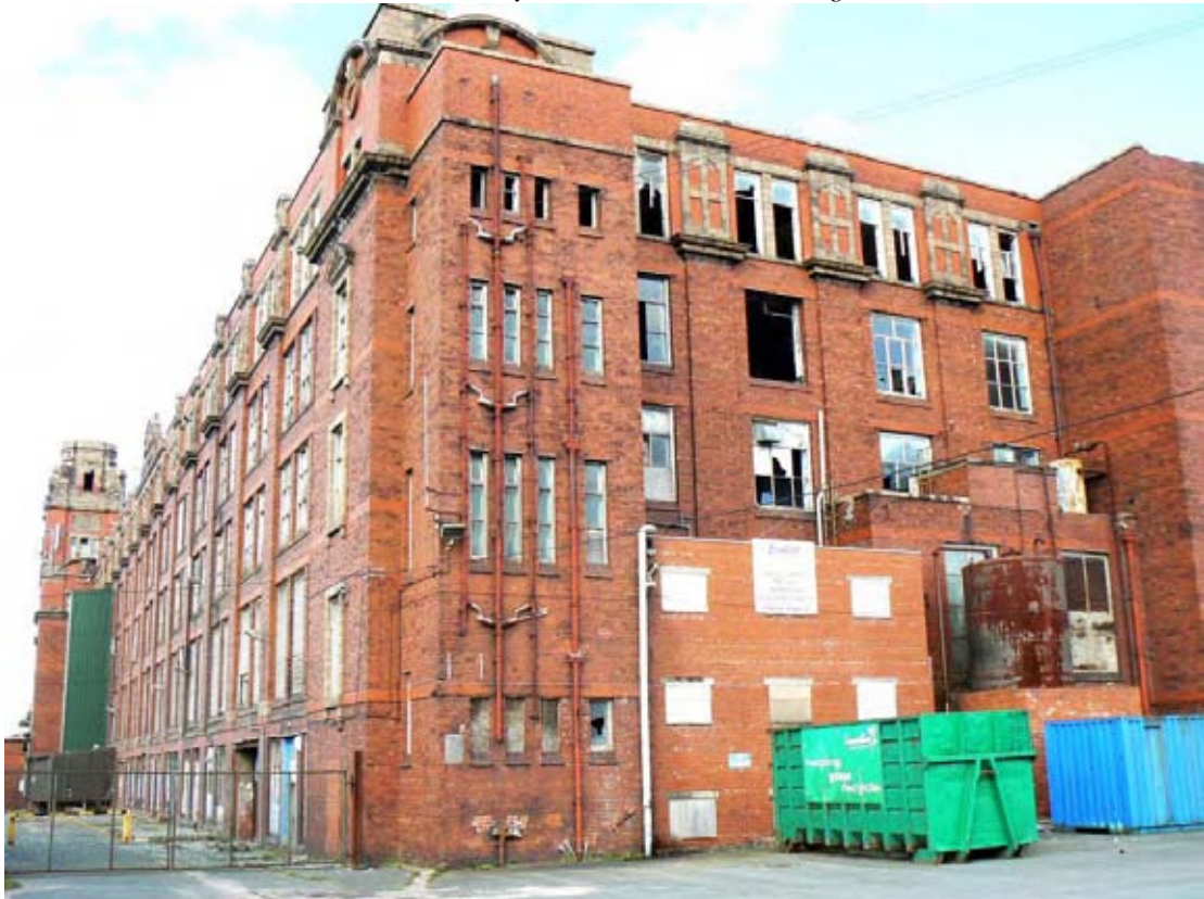
Plate 24: Wesley Street Mill, Bamber Bridge
