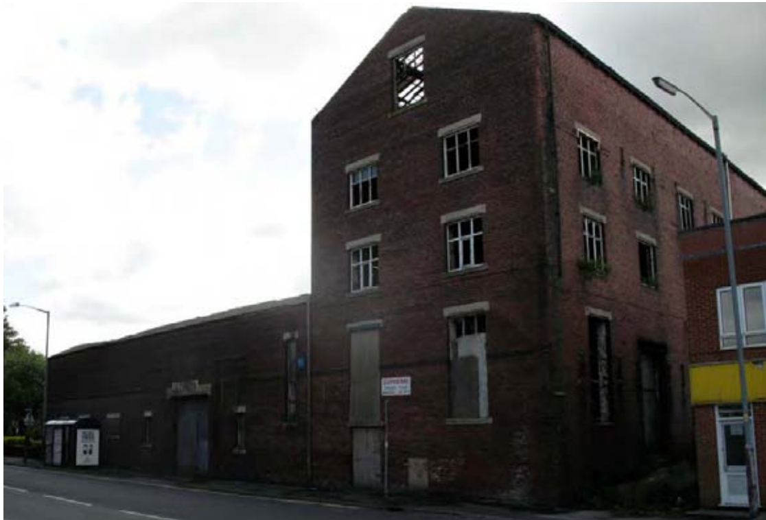
Plate 10: The derelict Globe Chemical Works, Church
