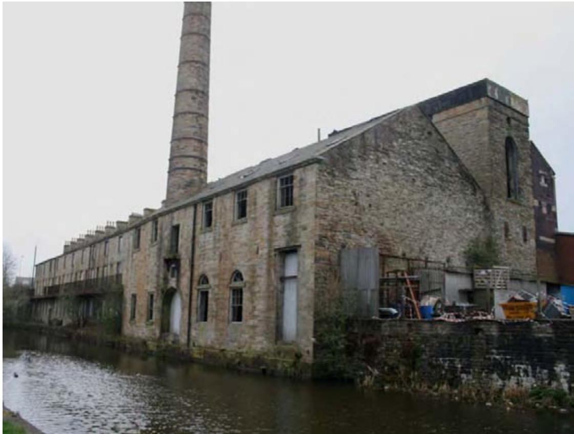
Plate 4: The derelict Sandygate Mill, adjoined by workers' housing on Slater's Terrace
