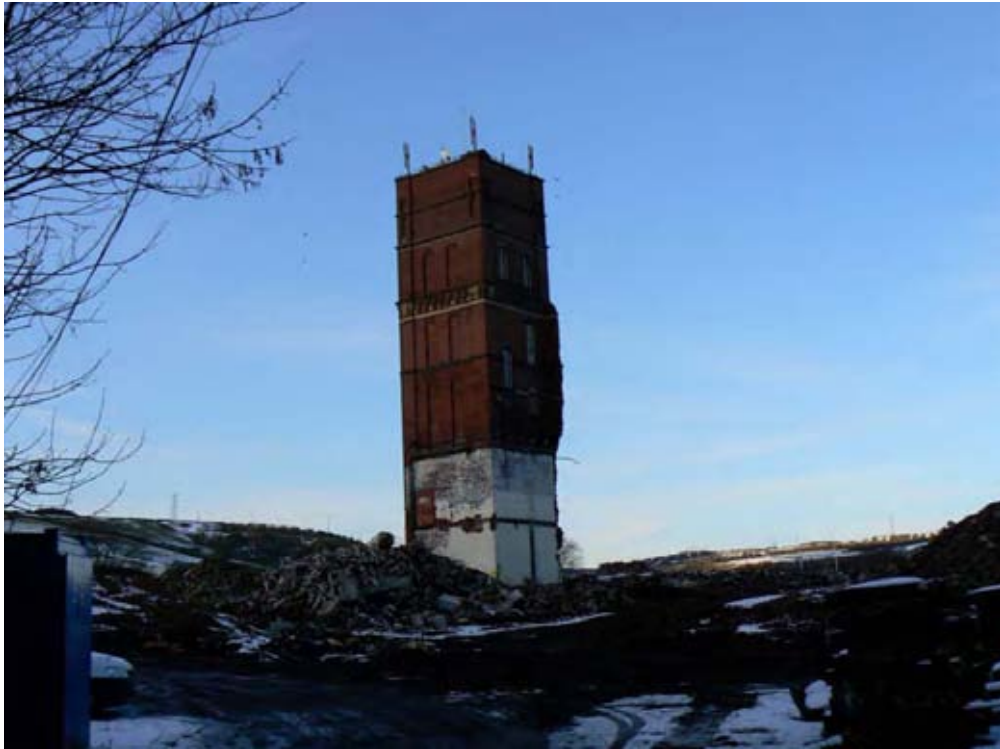
Plate 25: Orama Mill, Whitworth, during demolition in February 2009
