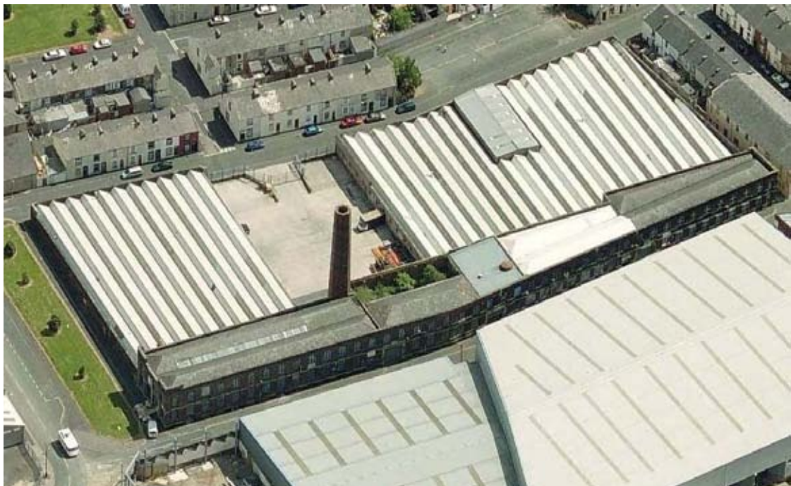
Plate 5: Elm Street Mill, Burnley, established in the 1880s as a room-and-power weaving mill
