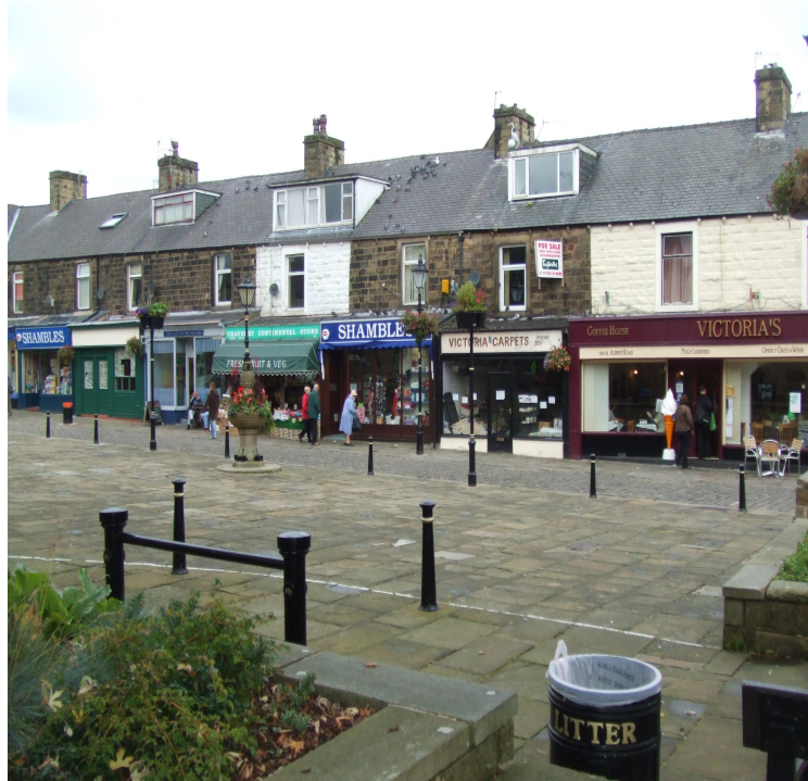
Figure 2: The Town Square on Albert Road
