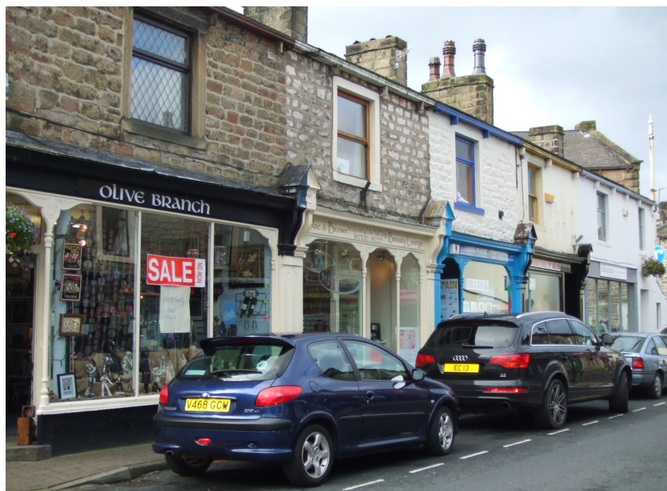
Figure 3: Traditional shopfronts on Rainhall Road
