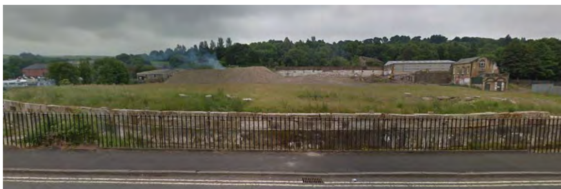
Figure 2.26: Existing site Viewed South from Spring Gardens Road CNDP6/16
