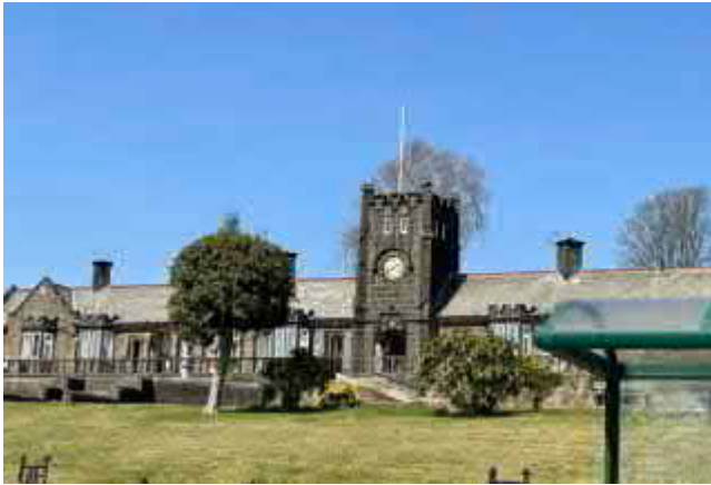
Hartley Homes Almshouses, built by the jam company founder, Sir William Pickles Hartley
