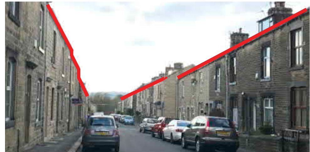
Figure 46: Uniform rooflines example within Colne
