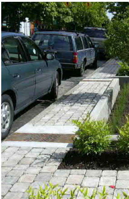
Figure 66: Precedent on-street parking
