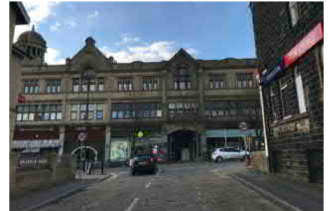
Grade II Listed Norway House and Old Co-op building
