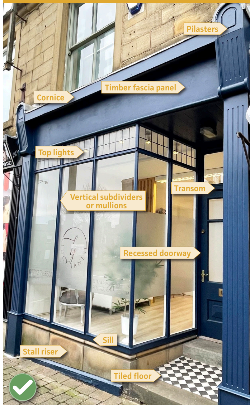
An example of a conservation aware shopfront at Lucy Janes
