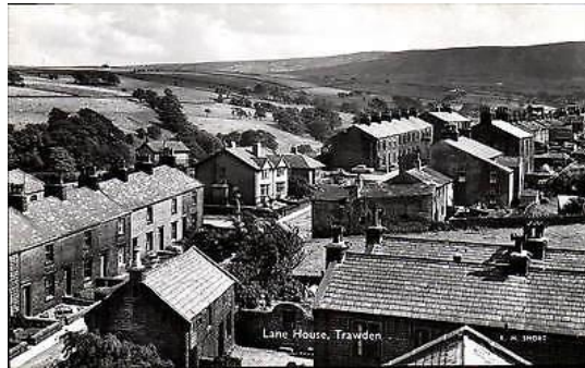
Lane House from the Church Tower
