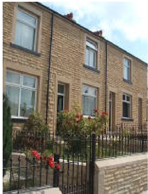
Block Improvements on Leeds Road
