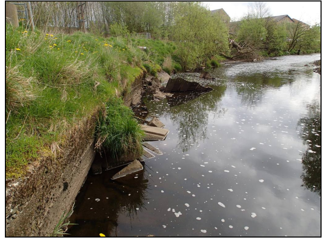
Photographs 14 & 15: Course of Pendle Water looking west and east. Erosion of the riverbank had broken concrete headwalls and sheet piles.
