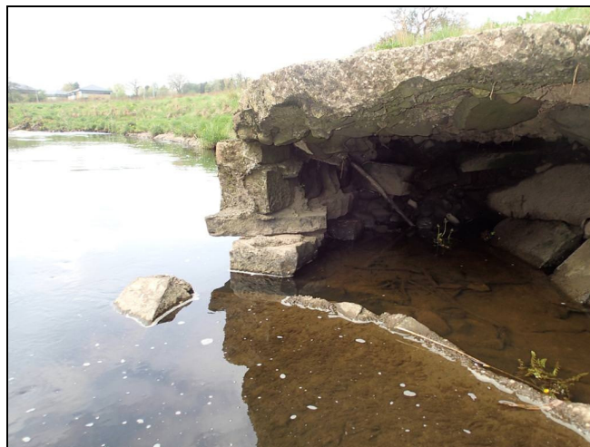
Photographs 16: Erosion of the riverbank had broken concrete headwalls and sheet piles.
