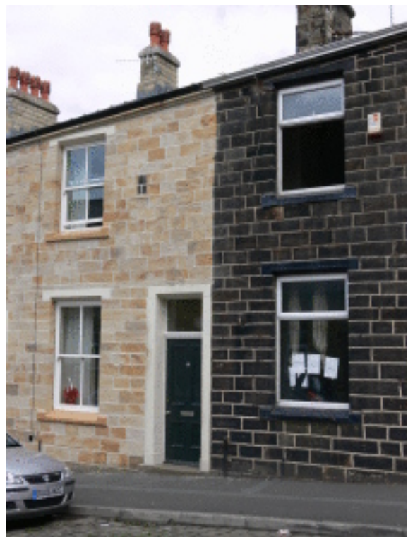
Picture A.7 Cleaned and uncleaned stonework in a terrace creating an inharmonious contrast
