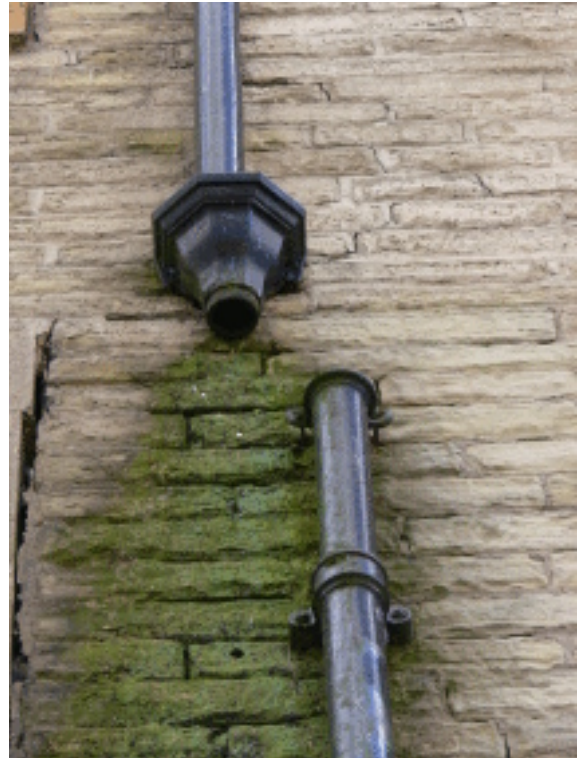
Picture A.1 Lack of maintenance can lead to problems
