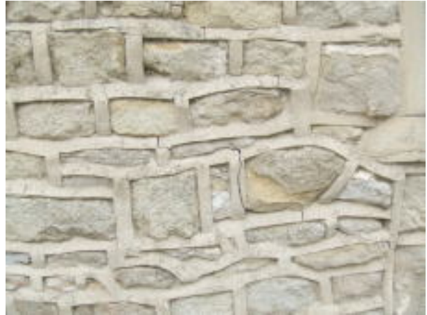
Picture A.5 Poor strap/ribbon pointing
