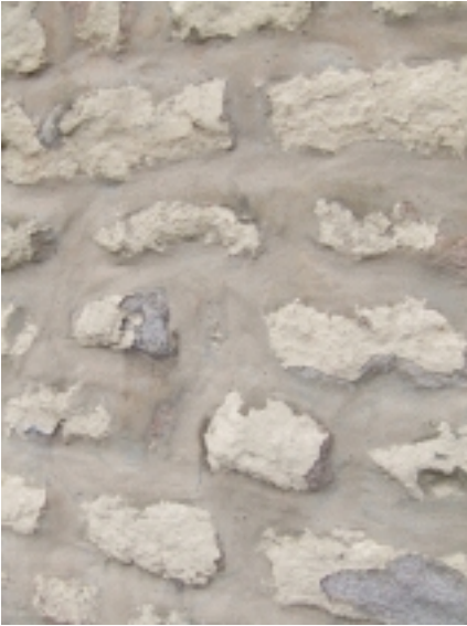
Picture A.4 Poor pointing, smeared across the stonework
