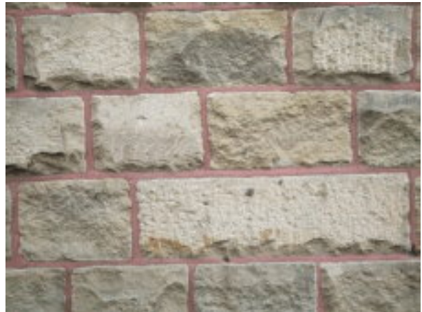
Picture A.6 Inappropriate mortar colour dominates the stone
