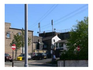
Two separate masts for antennae placed on an existing building above street level. The site is highly visible from the street below and the existing masts are not recommended for sharing.
