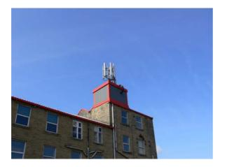
A medium size frame for antennae on top of an industrial building. The antennae are visible from the nearby road. This site is not likely to be suitable for sharing.
