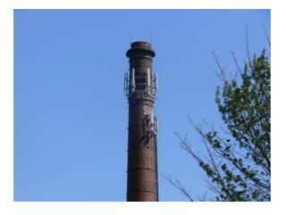
Antennae and dishes attached to an existing chimney on an industrial unit. The equipment makes good use of an existing building. Further antennae and dishes could be accommodated at this location, although consideration should be given to the impact on neighbouring uses, should land uses change in the future.
