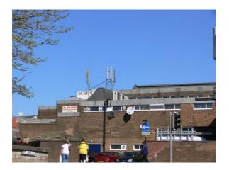
The mast and antennae are situated to the rear of the shop roof in Colne town centre. Three pairs of antennae are appropriately placed around the small tower. The antennae are visible from the street both at the front and rear of the property.
