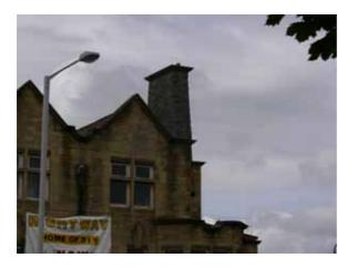
Four antennae are situated inside the chimney on the gable end of the former Greyhound Public House. The building is already a shared site with a further monopole and dish attached to another chimney (see second picture). The mast is a slimline design to reduce the impact on the surrounding area. Additional development is likely to be inappropriate at this site.
