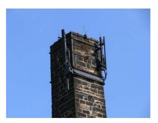
Antennae attached to an existing chimney which is visible from the nearby road. The equipment makes good use of an existing building. The site is suitable for sharing.
