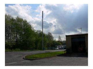
Telecommunication pole with antennae situated on an Industrial Estate. The mast is of a slimline design to blend in with the street lighting. This is a suitable location for a similarly designed mast.
